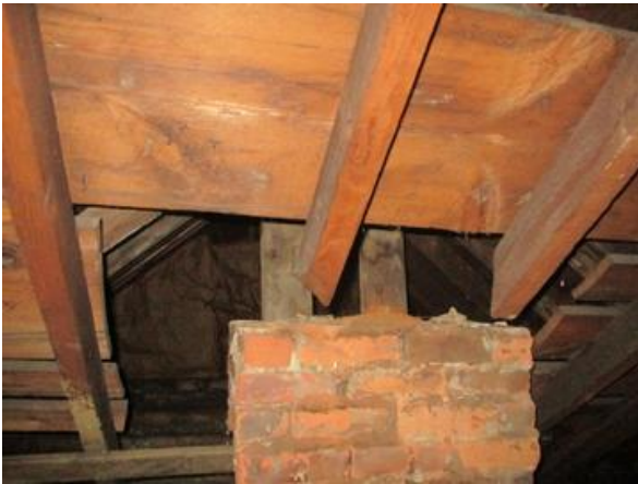
Rafter not fastened
