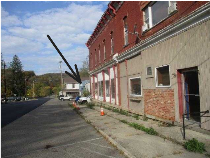
#15 Junk vehicles need removed on end of building.
