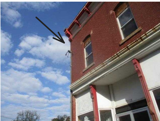
#17 Electric on left side terminated
