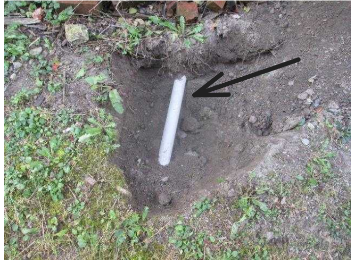
#2 Current water line coming from our building to the neighboring building
