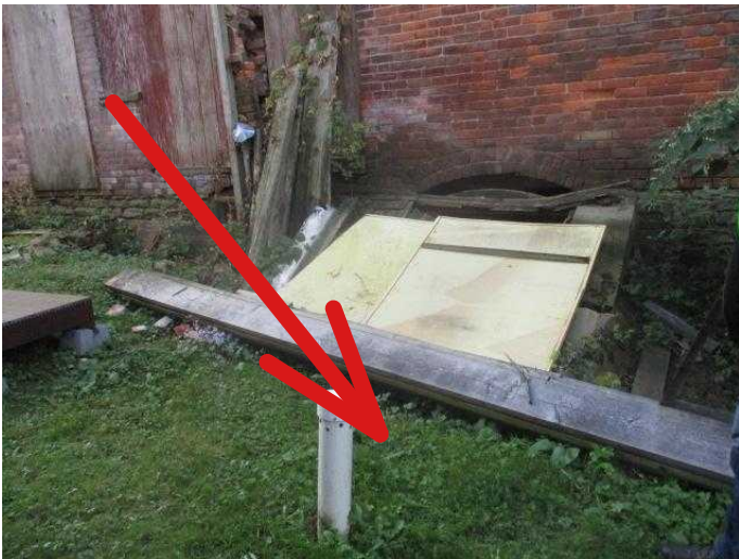
#9 Second sewer line will be terminated here
