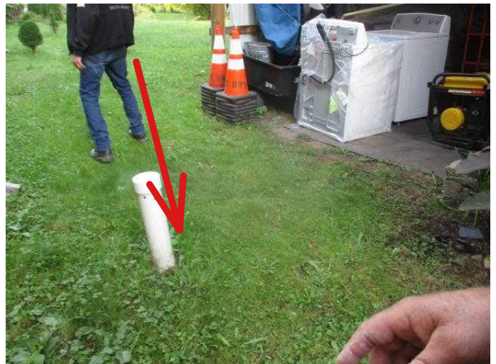
#6 Sewer drain will be terminated here
