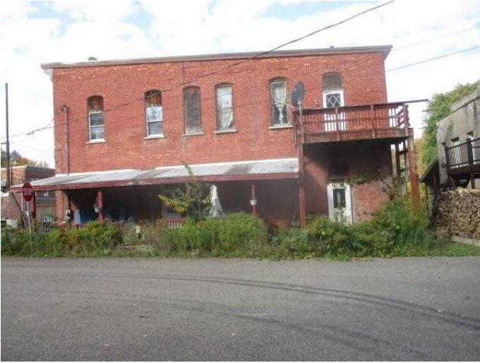
#1 Right side of the building
