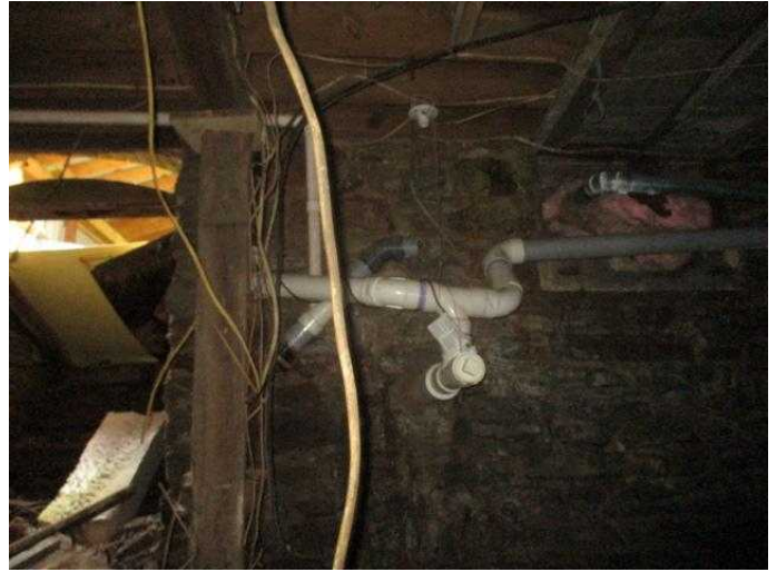
#32 Sewer in basement
